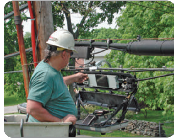
Installation of a Weather-Tight Aerial FOSC
