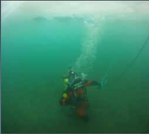
Diver under frozen Kvichak river placing fiber on river bottom
