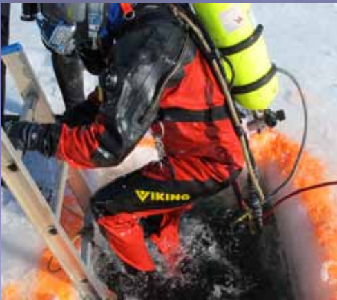
Diver under frozen Kvichak river placing fiber on river bottom
