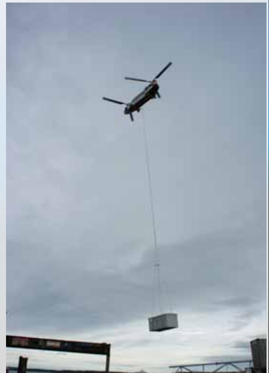
Chinook helicopter air-lifting power shelter
