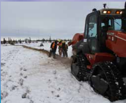
Fiber trench being dug near Igiugig, AK
